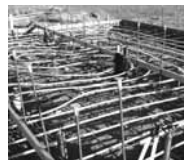
Radiant Floor Heat (under construction)
