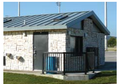
Concession space entry and roll-up curtain window.
