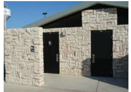
Restroom entry with louver/ screen vent above.
